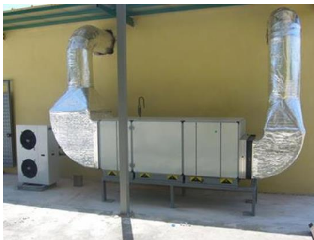
Figure 2. Air-conditioning unit, suction and pressure channels
