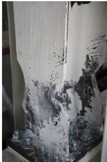
Fig. 9 Failure mode at 0.07 rad rotation [11]
