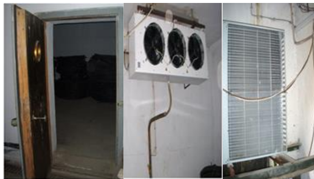
Figure 2. Cooling system elements
